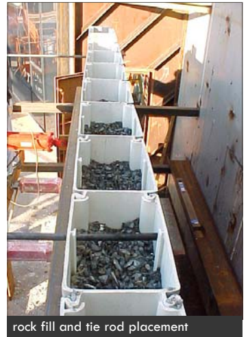
rock fill and tie rod placement
