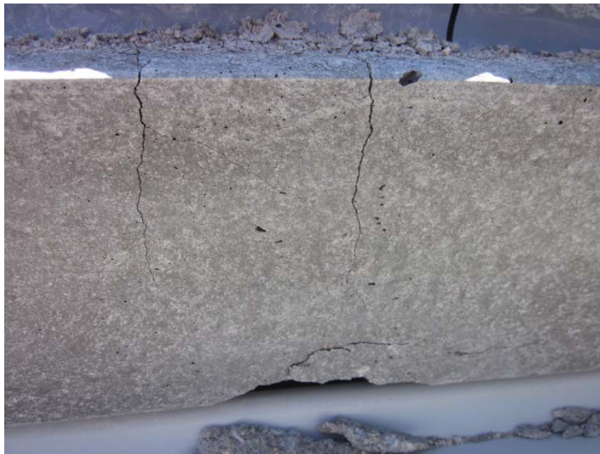
Photo No. 4 Typical Cracks in 8" Thick Specimen after Testing (End Cover Removed)
