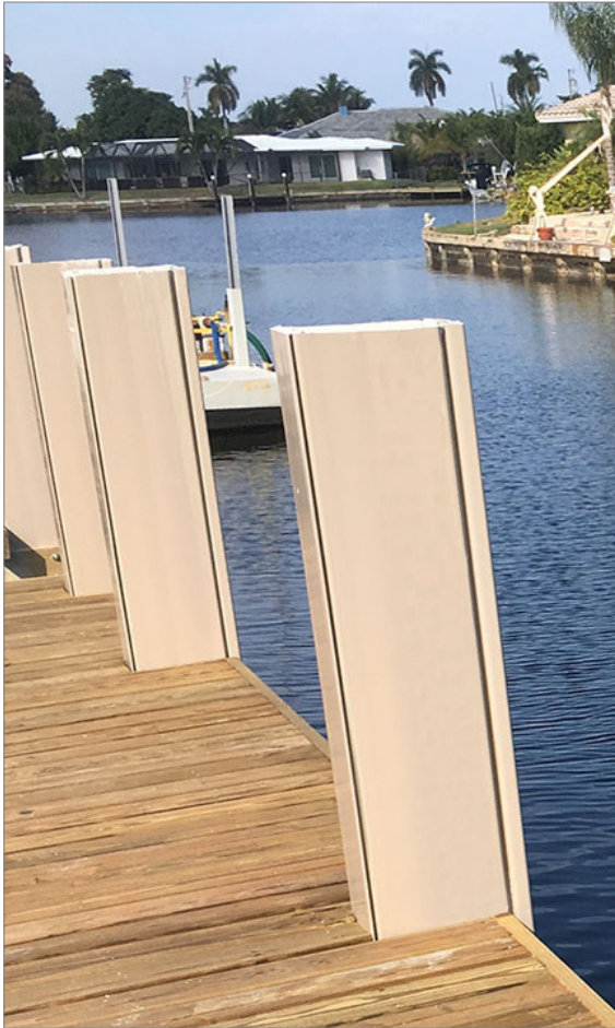
Truline dock piles shown above and below do not have top caps installed yet.
