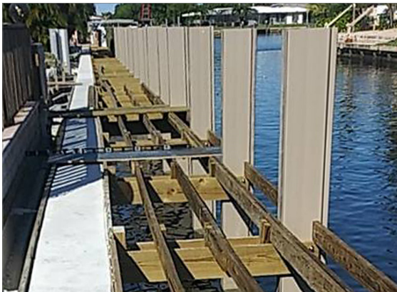
Truline dock piles shown above and below do not have top caps installed yet.
